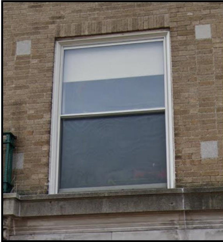
Above: Detail of Brick Molding prior to window replacement
